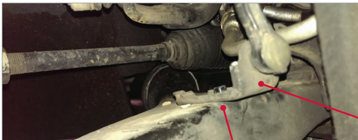
Figure 1: Rivet placed into arm, creating a mounting point for bolt
